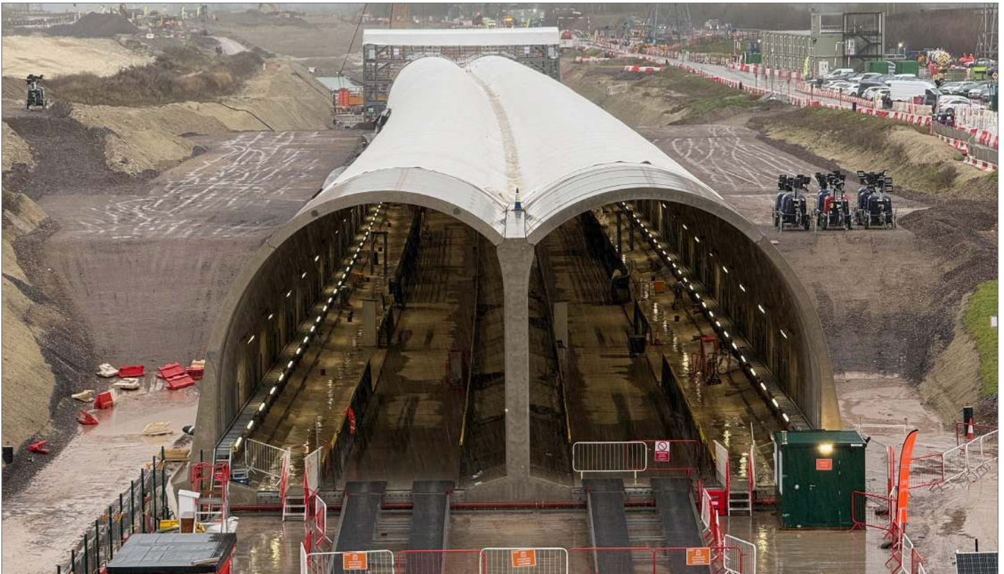
This photo, taken by Murray Cooke, shows how sections of the green tunnel are backfilled with crushed rock after a layer of waterproofing is fixed to the assembled pre-cast segments. The backfilling needs to be very carefully managed as it ultimately adds greatly to the strength of the structure.
