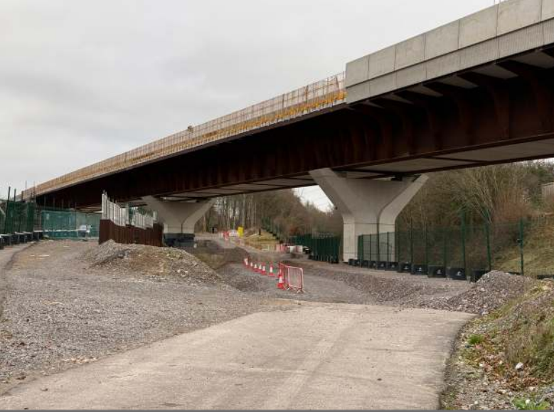
Small Dean Viaduct with parapets installed, giving an early impression of how the viaduct will look when they are installed over the main road. Photo: Murray Cooke
